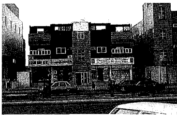
13 Riyadh (before) & 14 (after). Ground floor apartment transformed into commercial space
