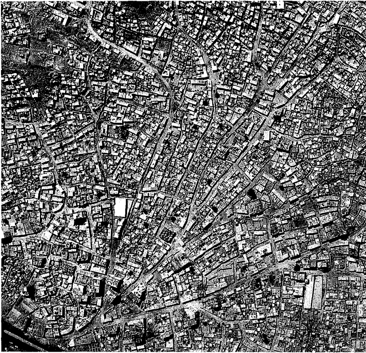
4 17 Al-Hindawiyah quarter, Mecca. The roads' and pathways' morphology are influenced by the mountains surrounding the site as constraint (courtesy of King Faisal University).
