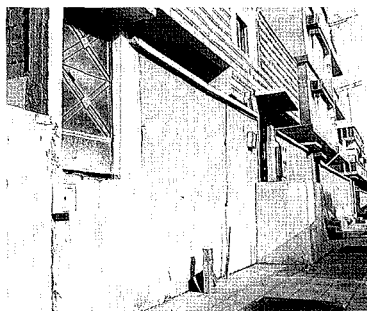
8 65 A fence in al-Khobar that was raised after the street level was raised only to be raised once more when the municipality repaved the street without removing the first layer
