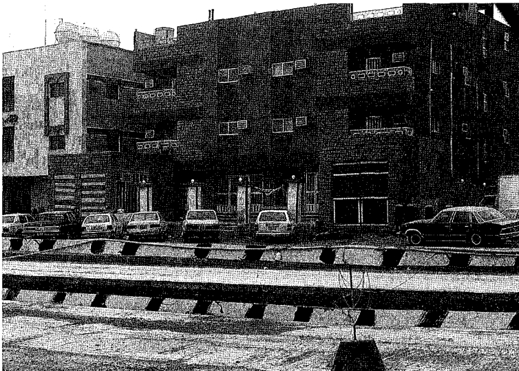
85 An owner of an apartment building decided to change his ground floor to commercial space. According to the municipal regulations he had to demolish the walls of the front yard and he did so. It is difficult, however, to demolish concrete columns, so he transformed them into lamp posts.
